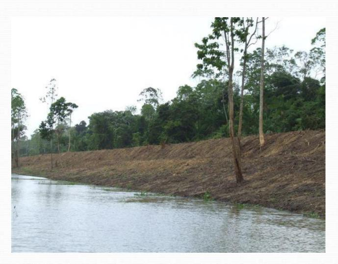
Piece of the canal bank of the Corantijn Canal washed away
